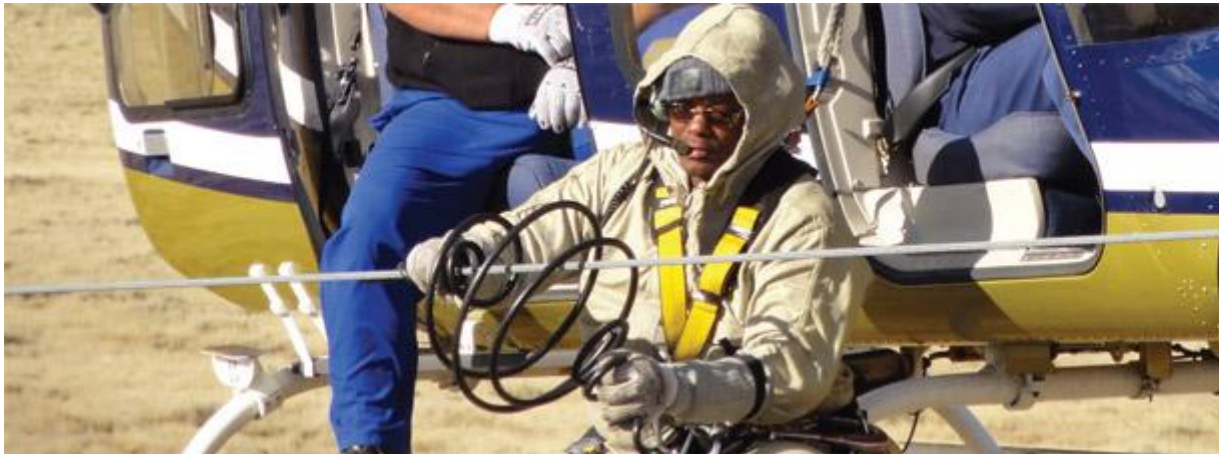
Bird diverters are strung on high-voltage power lines by helicopter
